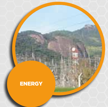
Furnas Electric Power Plant, Brazil.
